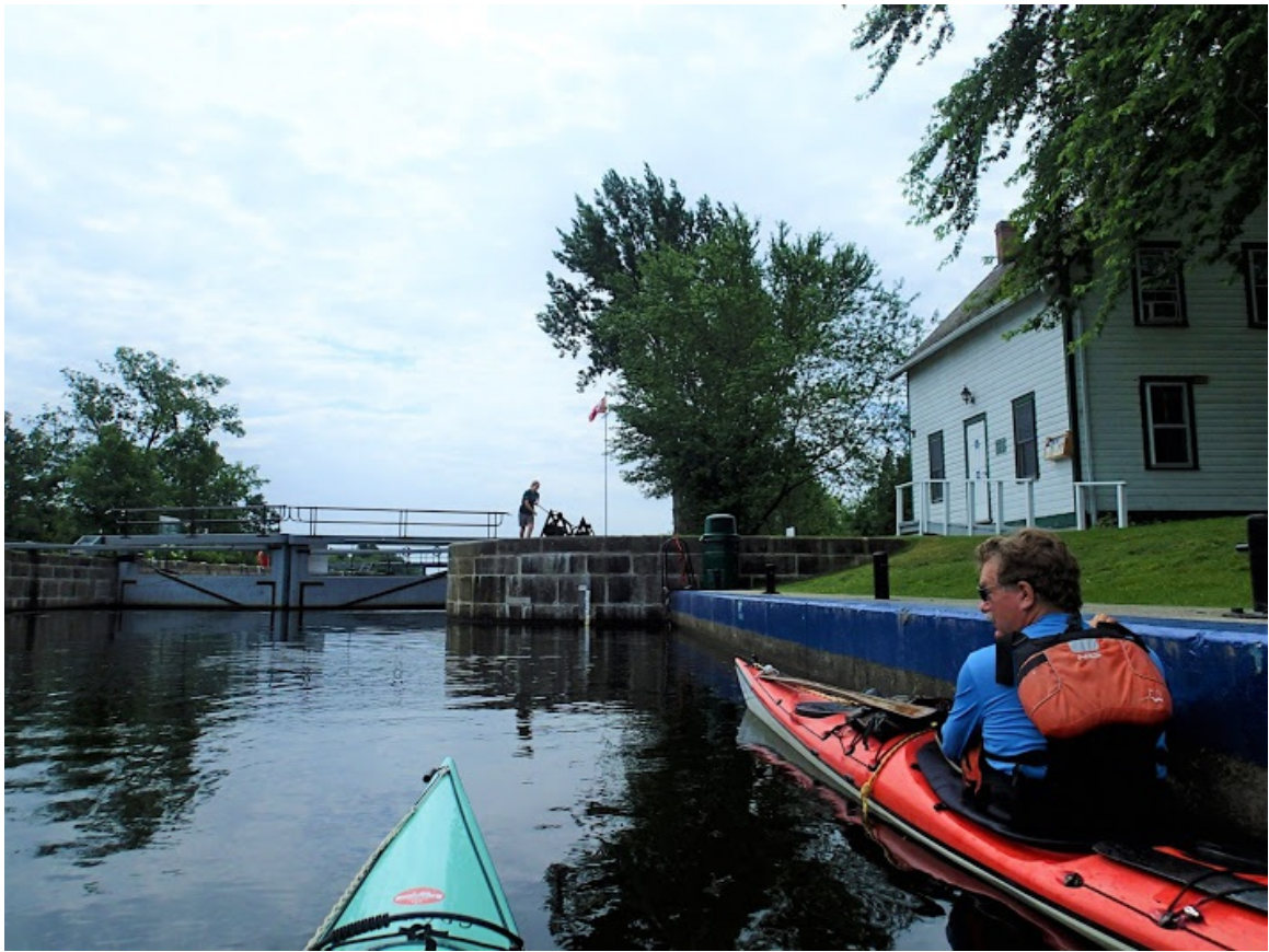
Waiting in the "Blue Line" at Smiths Falls. Credit: Ralph Heimlich.
