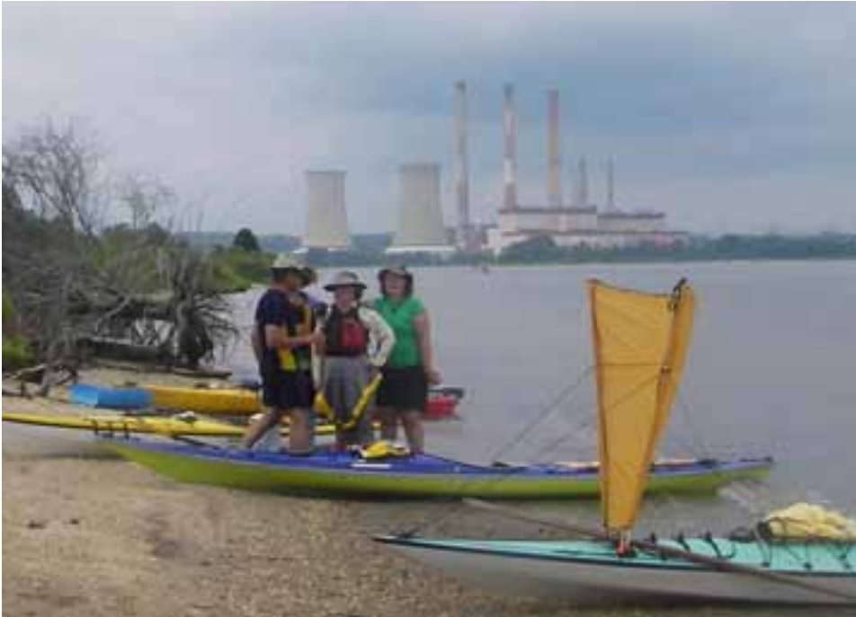
Chalk Point Power Plant.
