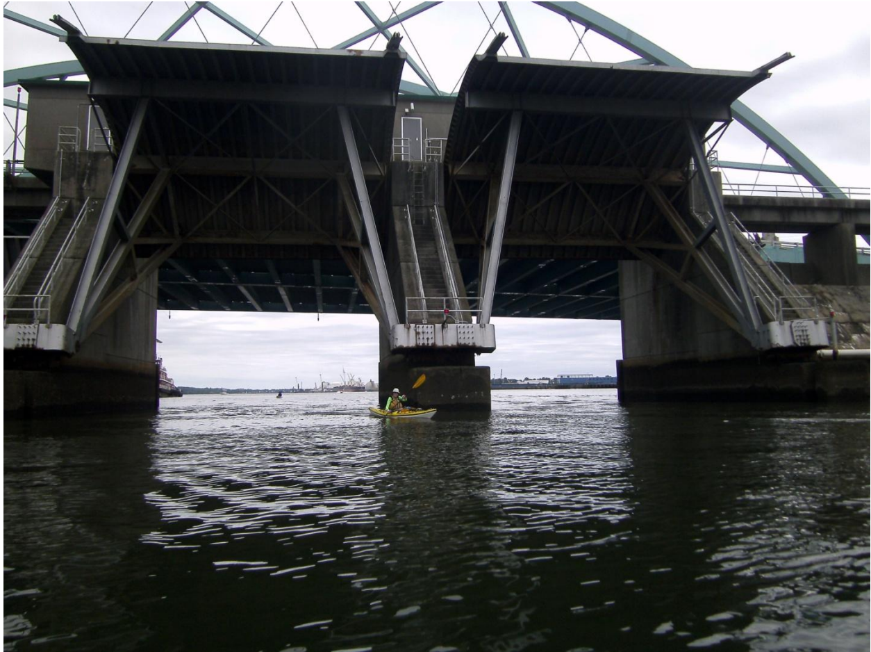
Figure 6 Providence Hurricane Gates and tugs
